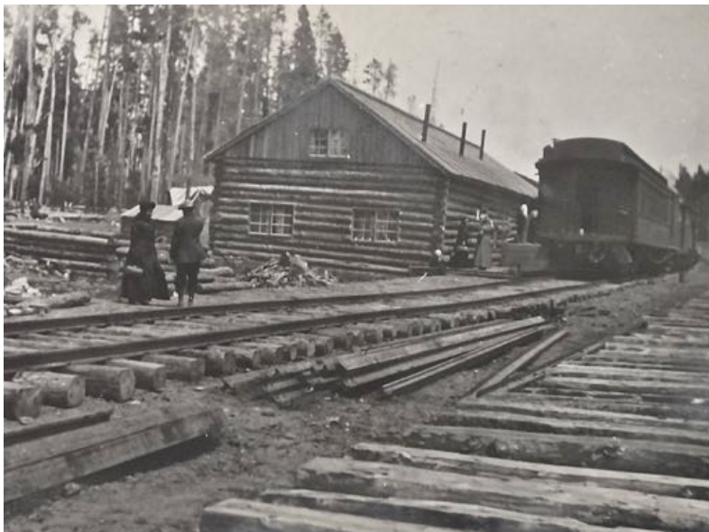
Tracklaying at Fox Park, Wyoming, near the log railroad depot. The photograph for this picture post card was taken in 1910 or 1911. This section of Wyoming’s Medicine Bow Mountains was a major producer of railroad ties in the U.S. in the first half of the 20 th century. (Source: Eric Miller.)
