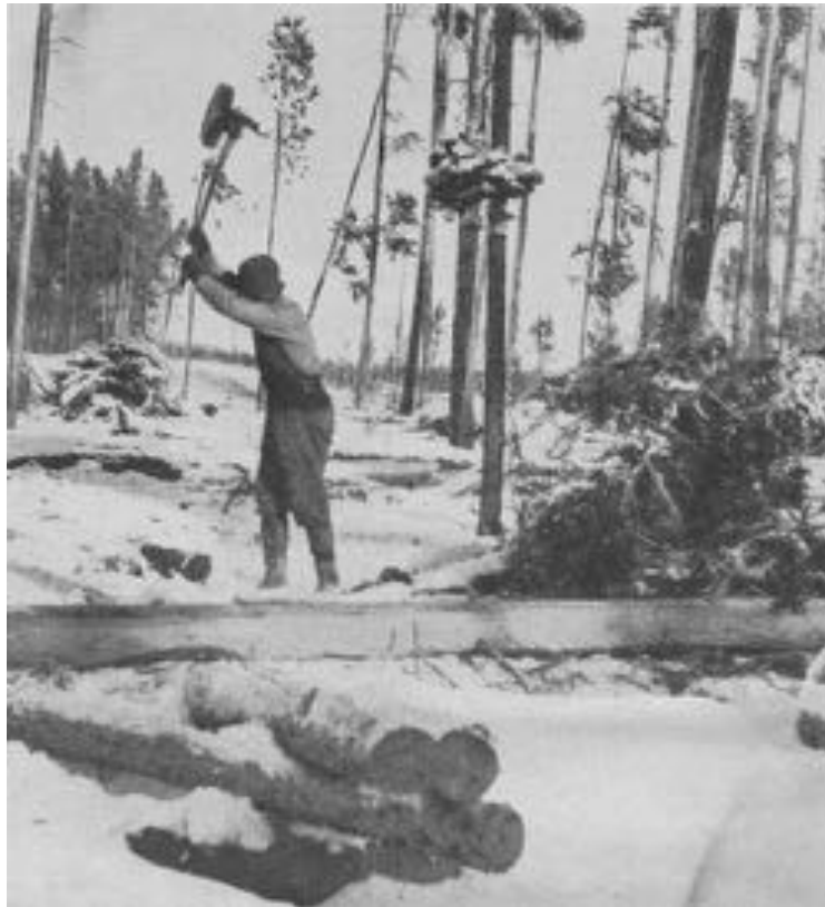
A tie hack hewing a railroad tie with his broad axe in the Medicine Bow National Forest (Source: U.S. Forest Service)
