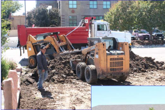
Step 1 (Above and right) Completely tear out the old parking lot in front of the annex and prepare the dirt base.
