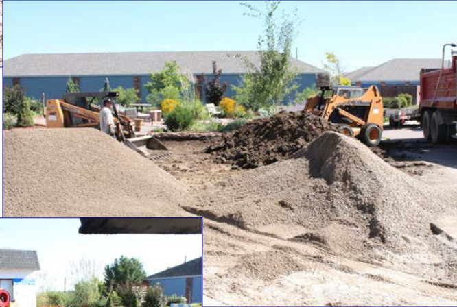
Step 1 (Above and right) Completely tear out the old parking lot in front of the annex and prepare the dirt base.
