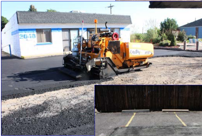
Step 2 Put down the paving.
