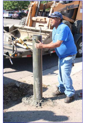
Step 4 Install stanchions to link chains to keep large trucks from turning around in the parking lots. This has caused problems in the past.
